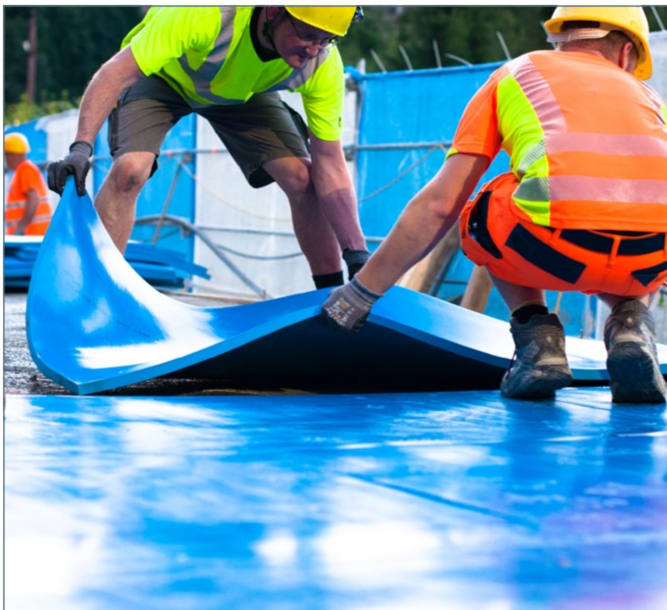
Installation situation of elastic support in the track bed
